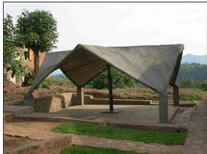
Photo: Thin-Shell Concrete Kitchen at L'Esperance Orphanage, built by local workers and Birambye.
